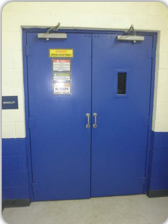
Double swing fire-rated doors
